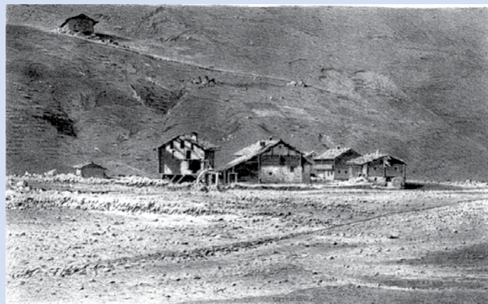
Fig. 60: Photo of the sand-covered valley plain near Vals shortly after the flood and the following debris flows 3 (see p. 32).
