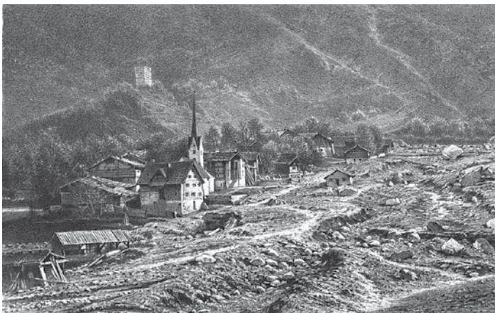
Fig. 54: Floods and debris flows in Zignau (left) in 1868 35 and 1987 (right).
