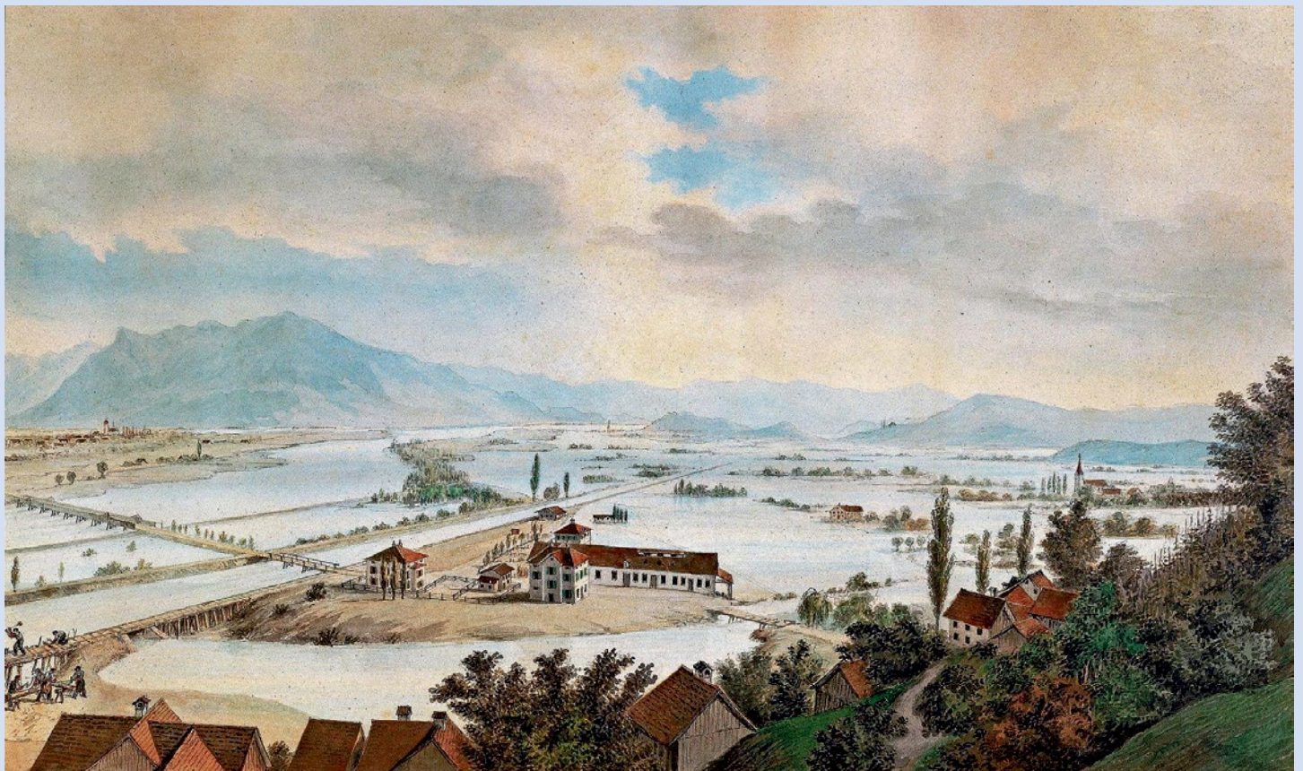
Fig. 28: The flood of 1868 by Au (St. Gallen) 1 (watercolour). On the left, the damaged train bridge is reproduced. This very reliable and modern picture is a significantly better illustration of the extent of flooding in the Rhine Valley than any written source, especially when it is combined with close-ups such as the early photography from Lustenau (Fig. 1, on the watercolour, left in the background). However, based on the start of repair works, it remains unclear if the picture reproduces the highest water levels or an already reduced water level.
