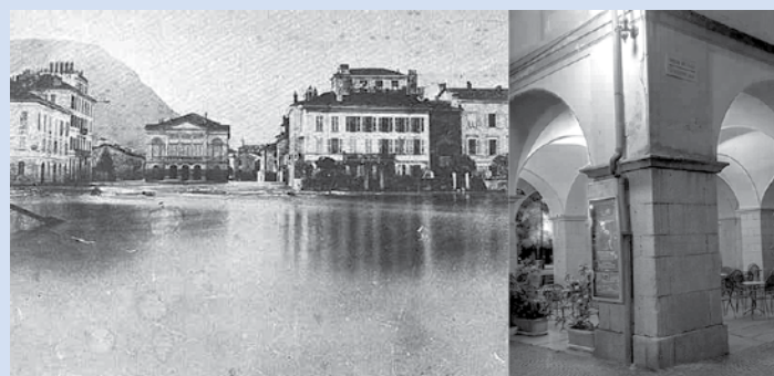
Fig. 5: Flood of Lake Maggiore in Verbania 1 in 1868 (left). At the time of the highest level, the water reached over the arcades of the old town houses (flood mark in the photo on the right).
